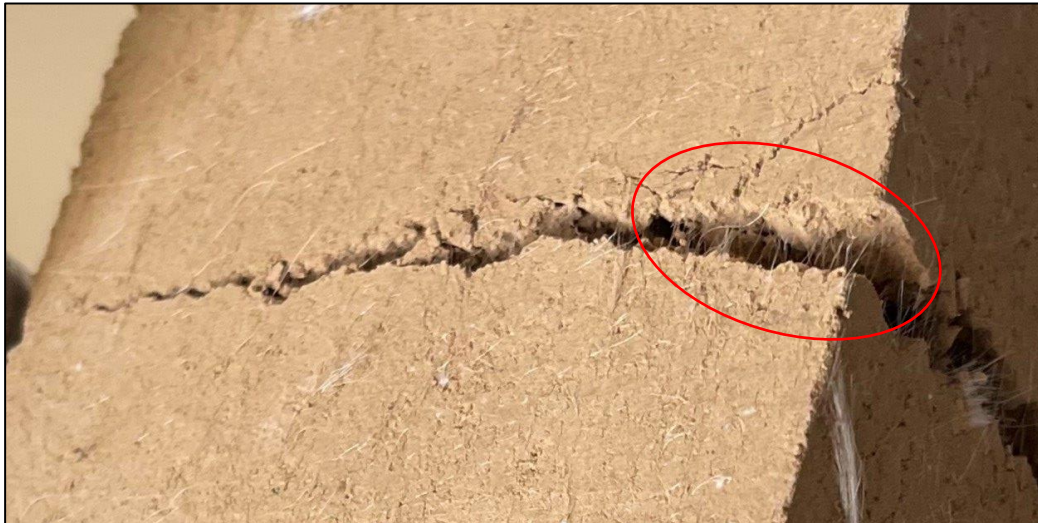
Fig. 15. Fibers bridging crack during the flexural test.
